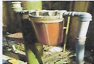
Plate 4.4. A borehole filter stained red from suspected iron oxide in Ozoro. Source:Fieldwork.
